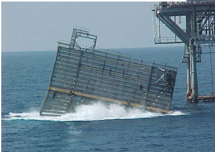
Figure 7 – Platform topples on location
