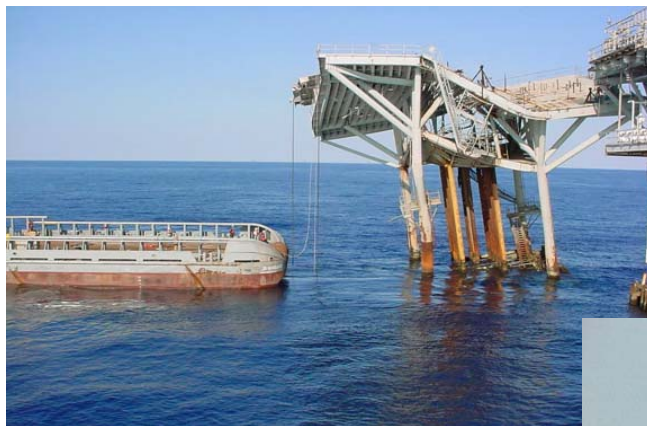
Figure 5 – Toppling rigging connected
